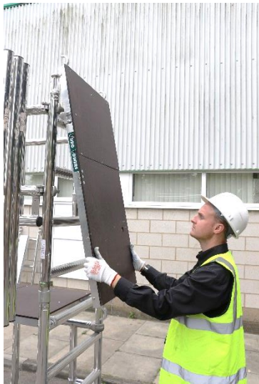
16. The platform can be located on the opposing side of the tower from the frames.
