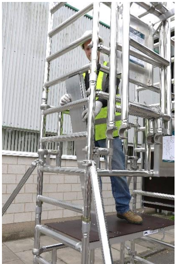
26. Temporarily locate the toeboard assembly on the platform to allow access to the additional platform that is stowed.
