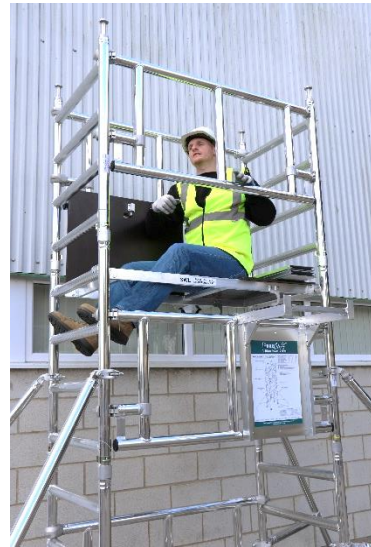
13. Fit 2 guardrail frames, with the top hook (facing outwards) set above the top rung of the frame.
