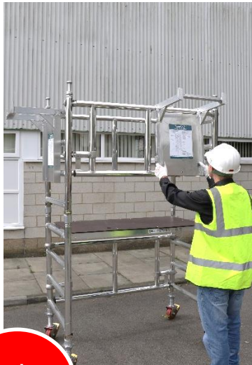
11. Remove toeboard and fit 2 assembly brackets in the position shown (side and front)
