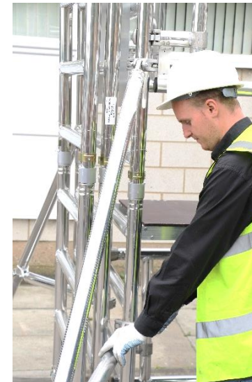
19. Fit 4 stabilizers, one on each upright of the tower.
