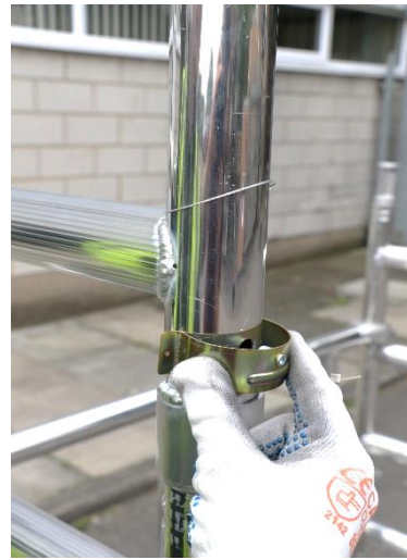
13. Engage interlock clips.
