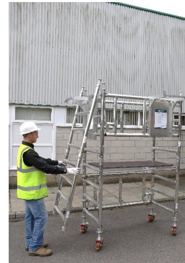
14. Stow 4 frames (2 pairs) on the side assembly bracket.
