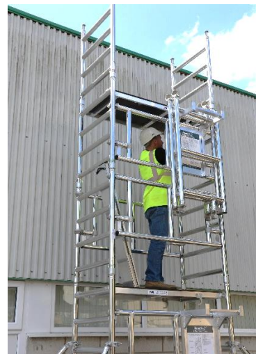
27. Fit the platform, 1 rung above the side frame location as shown.
