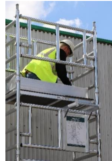
14. Fit toeboard by unfolding the set above the platform (please use labelling as a reference to ensure that the toeboard is the correct way up).
