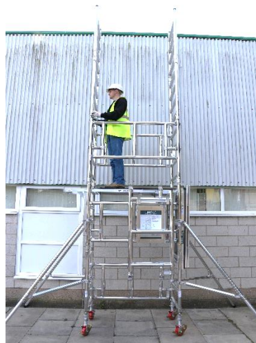
18. Repeat this process for the opposing side, ensuring that all interlock clips are engaged.
