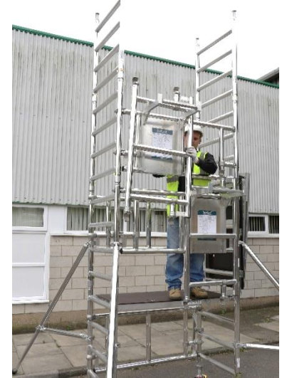
25. Retrieve a side guardrail frame from the front assembly bracket and locate it as shown.
