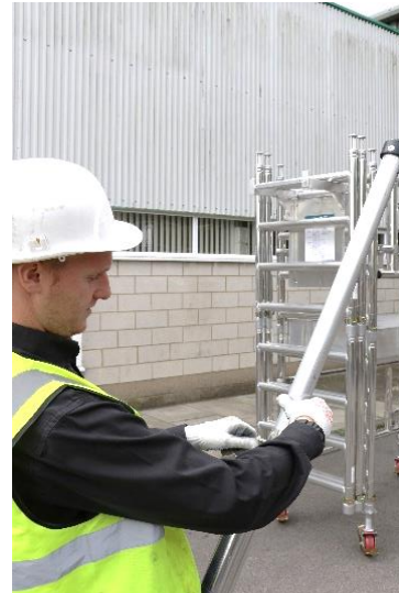
18. Before fitting stabilizers, release the pin to enable extension.
