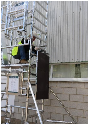
26. Remove the remaining platform from the lower section of the tower and pass up through the side frame.
