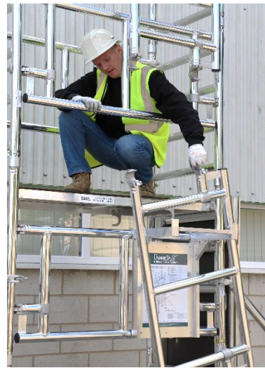
23. Retrieve 2 stowed side guardrail frames from the lower assembly bracket (front) pass them up to be relocated on the higher assembly bracket.
