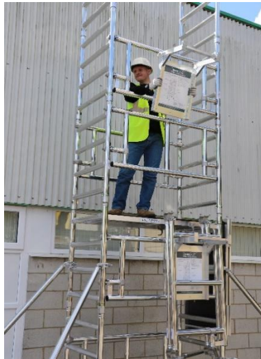
22. Place the removed bracket on the top rung of the tallest guardrail frame as shown.
