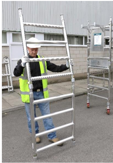
12. Assemble the frames in pairs as shown.
