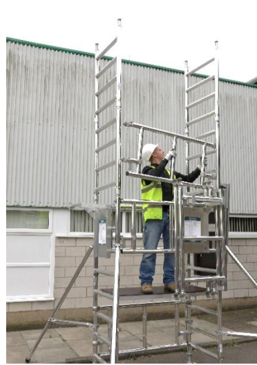
23. Retrieve a side guardrail frame from the front assembly bracket and locate it as shown.
