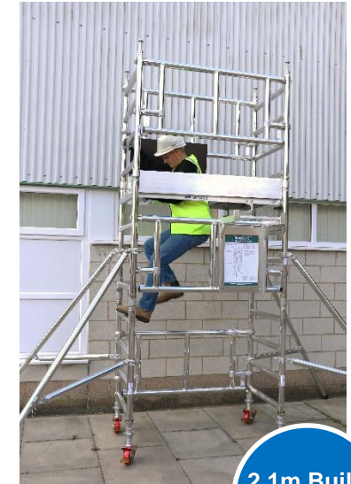
15. Access the platform using the trapdoor as shown and begin work.
