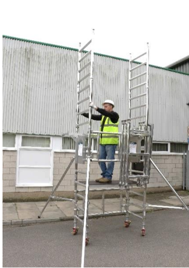
22. Repeat this process for the opposing side, ensuring that all interlock clips are engaged.
