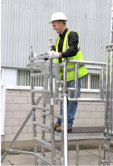
21. Retrieve a set of frames from the side assembly bracket and fit.
