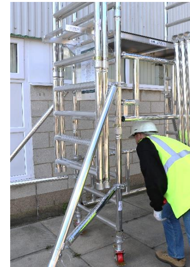
20. Access the platform by passing under the side frame and via the trapdoor platform.
