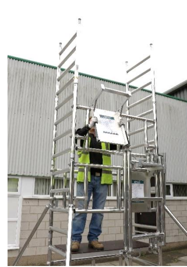
24. Relocate the side "empty" assembly bracket on the front of the tower (top rung of the tallest guardrail frame as shown)
