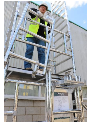
19. Retrieve a side guardrail frame from the front assembly bracket and pass upwards as shown.
