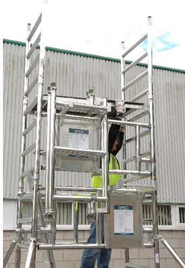
27. Fit the platform, 1 rung above the side frame location as shown.
